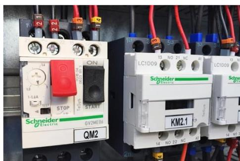
Gambar 4. 2 Overload Relay / Thermal Relay
