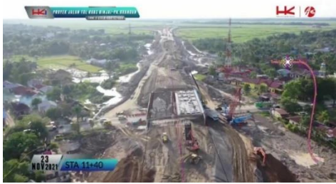
Gambar 3.1 Lokasi jembatan underpass STA 11+140
