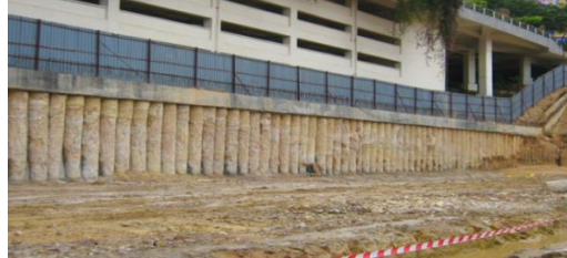
Gambar 9. Dinding Soldier Pile
