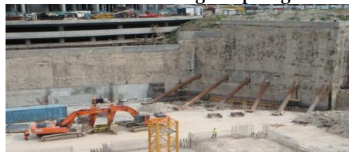
Gambar 7. Dinding Diaphragm
