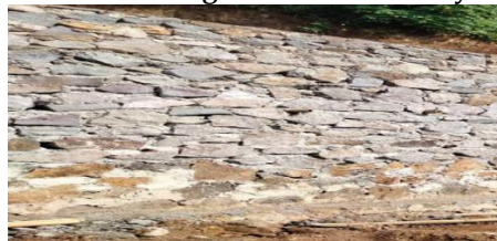
Gambar 1. Dinding Gravitasi (Gravity Wall)
